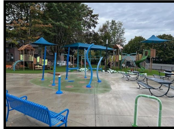
Las Casitas Park Under Construction
